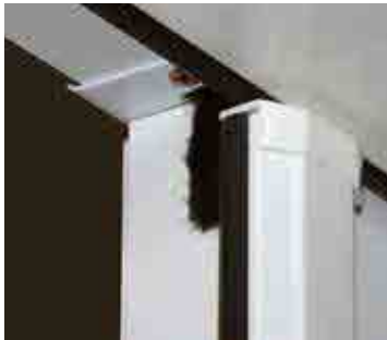
Astragal secures inactive door at top and bottom of your french door system
